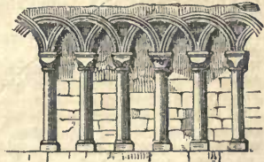
Interlacing Arcade, Norwich Cathedral.
